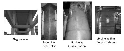
Fig.15 Real applications of Duplex Jacketing
